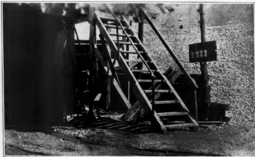
Outdoor Plug-in Station for Two Phase Motor Mounted on truck with Hoisting Used with Dragline Scraper.
